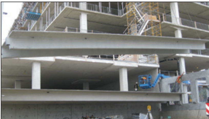
2010 Ontario Concrete Award winning project for Structural Design Innovation
