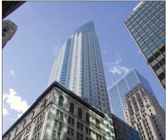
2005 Ontario Concrete Award winning project for Structural Design Innovation
