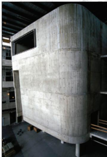
The entire floor of the 22,050m<sup>2</sup> facility has exposed concrete finish. The floors are either retroplated cast-in-place concrete or retroplated access flooring, providing Centennial a resilient, low maintenance surface. The ceilings have exposed concrete beams and columns throughout with acoustical tile infills. With the exposed concrete, it gave it an
