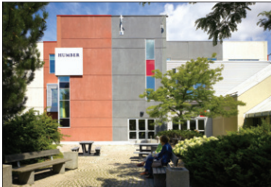
2008 Ontario Concrete Award winning project for Structural Design Innovation
