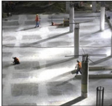
**Framing Systems:** the project utilized a combination of two-way slabs with tapered drops, one-way slabs on concrete beams and two-way slabs on concrete beams.
